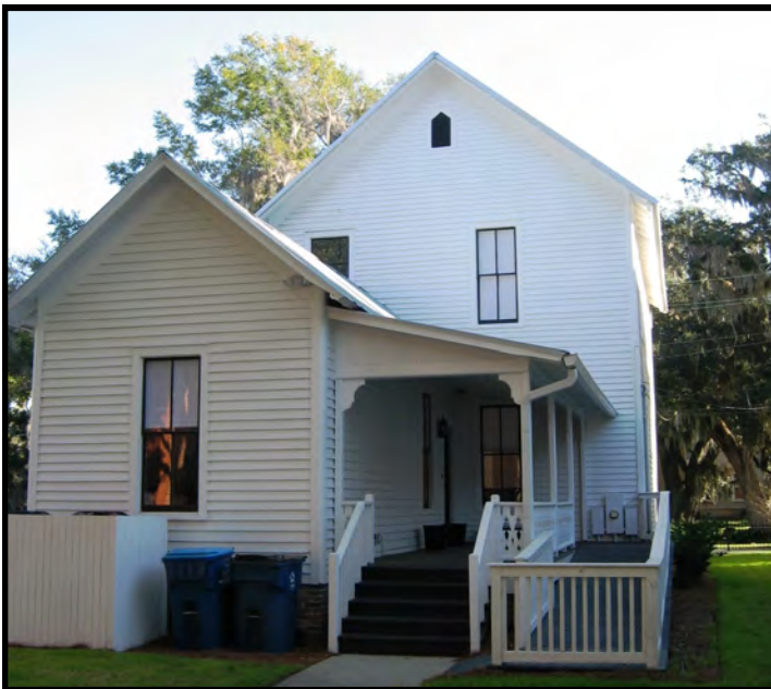
Example of an appropriately sited and designed ADA ramp at the rear of this dwelling (left and right). The ramp is consistent with the style of the dwelling and is not readily visible from the street.
