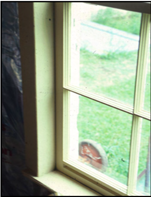
Replacement windows should be of wood, aluminum clad or a compatible alternative material. They should have true divided lights as illustrated above or simulated divided lights as shown below.
