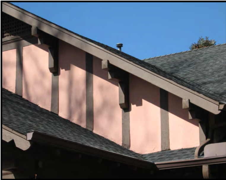
Exterior wall siding materials may also include half-timbering and other decorative designs (1008 Gordon Drive, SE).
