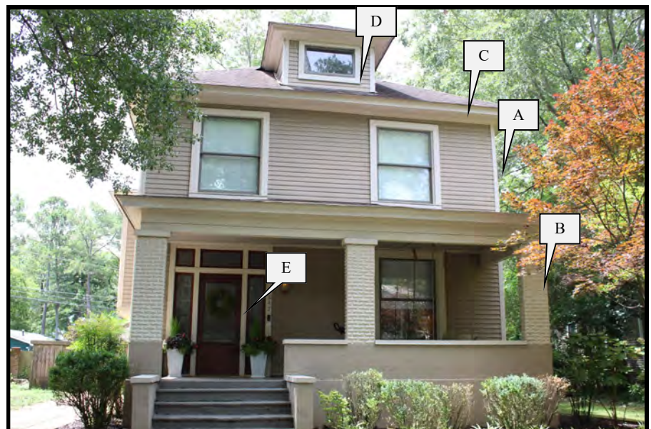
The American Foursquare at 845 Sherman Street, SE, has a full-width porch with rock-faced concrete columns on a brick railing.
