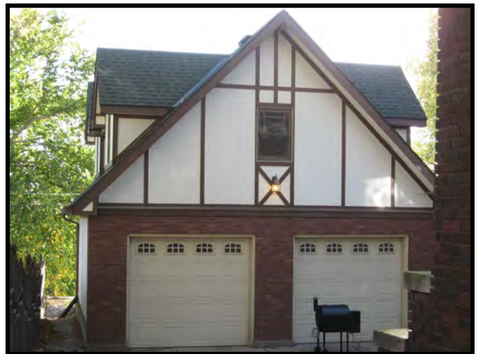
YES: This new garage was designed to be compatible with the Tudor Revival dwelling with its gable roof, exterior of brick and stucco and half-timbering.
