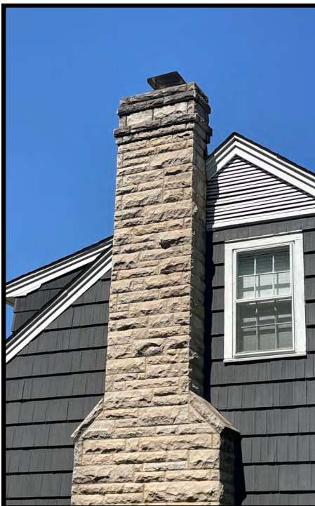
Corbelled brick is a common feature of chimneys on dwellings from the late nineteenth and early twentieth centuries (422 Jackson Street, SE).
