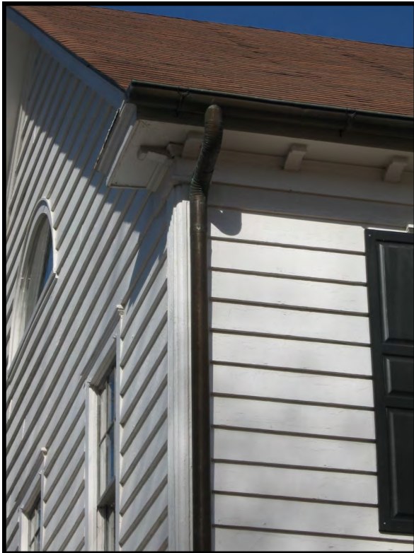
Gutters are recommended to be half-round design with round downspouts, (1006 Gordon Drive, SE, left and 305 Lafayette Street, NE, right).
