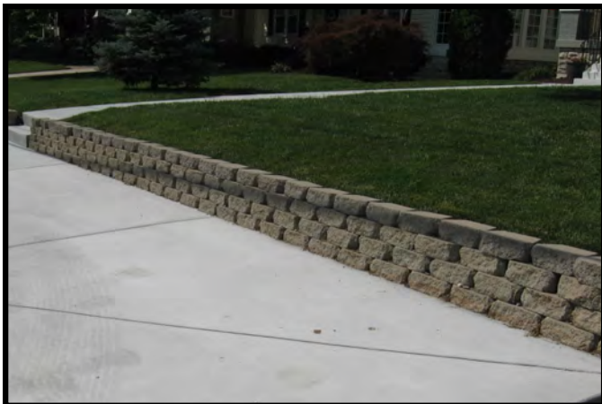
Retaining walls of non-traditional materials such as undersized concrete blocks (left) and split-face blocks (right) are not appropriate for the historic overlay districts.
