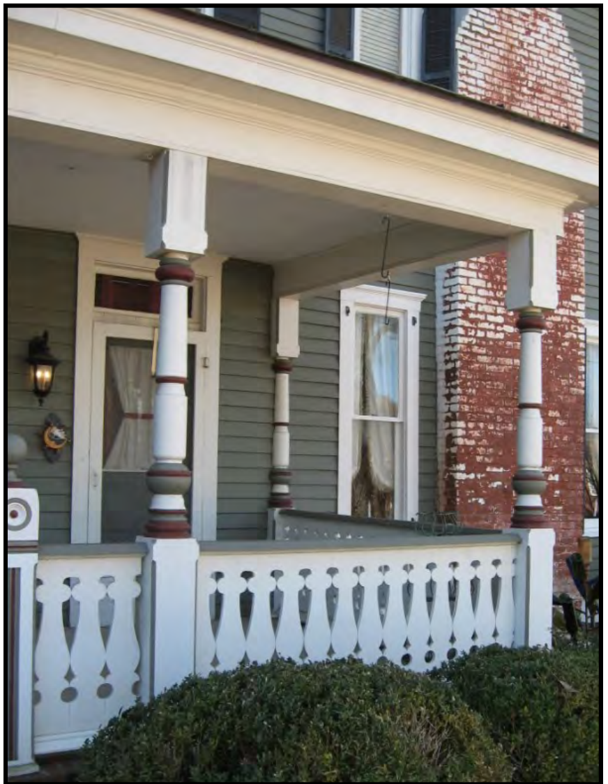
Milled wood porch columns and intricate woodwork on the porch railings are one of the most important defining features of a dwelling's style (618 Oak Street, NE).
