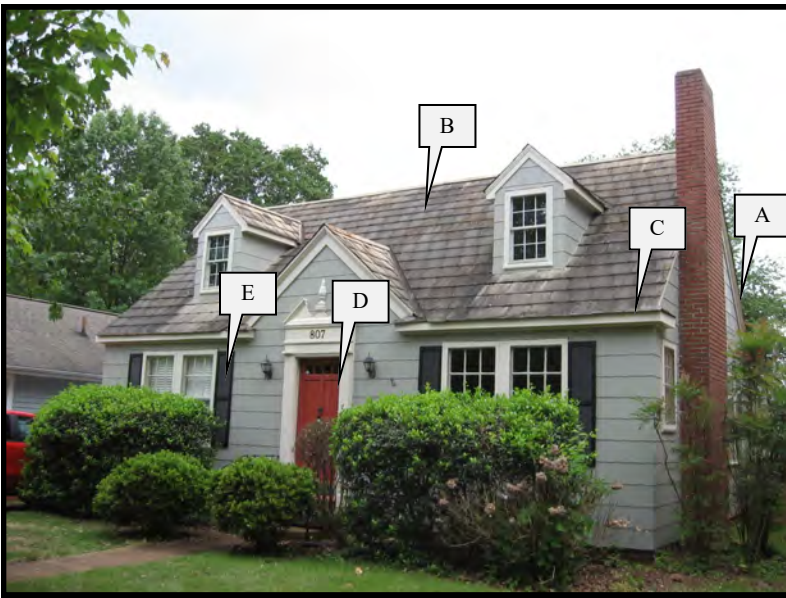
Minimal Traditional style dwelling with Colonial Revival influences at 807 Grant Street, SE.
