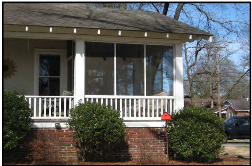
Screening of front porches is discouraged but may be appropriate if minimal structural framing is used (826 Gordon Drive, SE).
