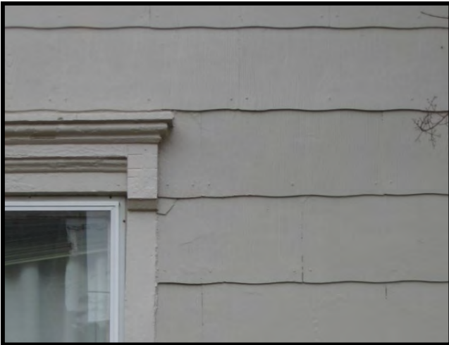
A number of dwellings in the historic district had the original wood siding covered with asbestos shingles in the mid-twentieth century as at 119 Lafayette Street, NE (above). Wood siding beneath asbestos shingles is often in good condition. After the asbestos shingles are removed, the siding has the potential for restoration (right).
