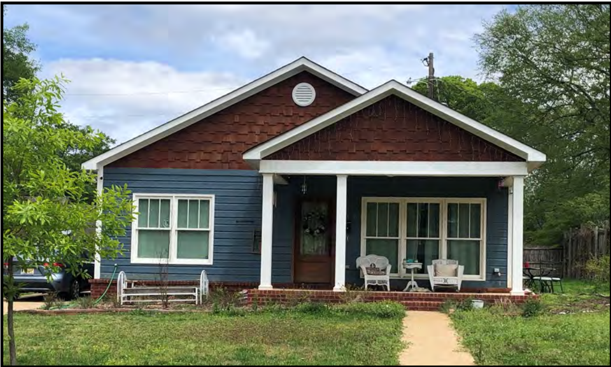
The infill dwelling at 217 Cain Street, NE, was designed with appropriate scale, materials and orientation to the street. The vertical upper sash windows are in keeping with the Craftsman style dwellings in the neighborhood.
