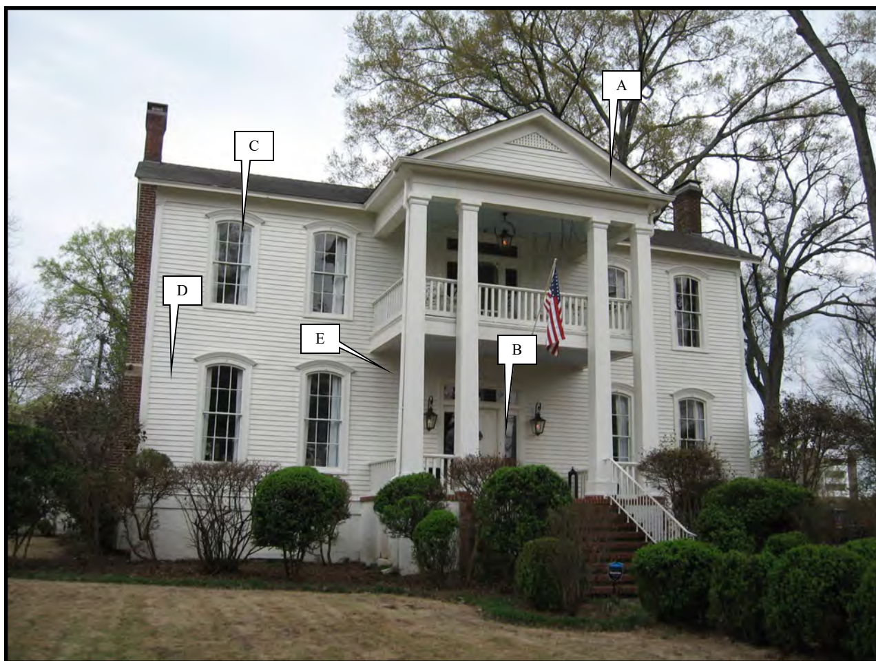
The Greek Revival dwelling at 504 Line Street NE, features a prominent, full-height portico.
