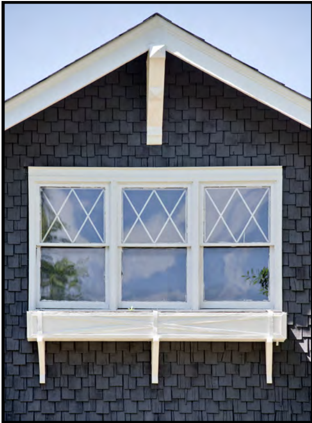
Architectural details include design elements such as diamond light upper sash windows and wood shingles (804 Jackson Street, SE).
