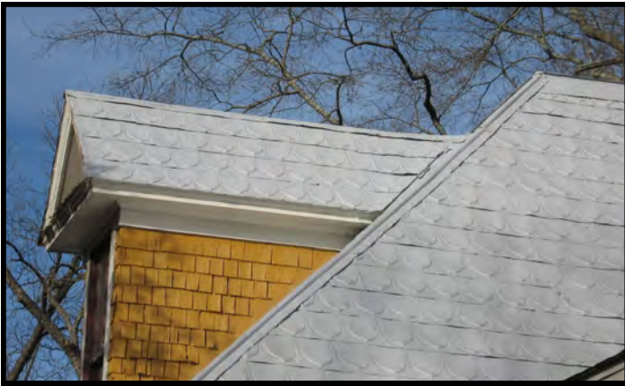
Several dwellings in the overlay districts retain original pressed metal shingle roofs which should be preserved and maintained (left, 644 Johnston Street, SE, and right, 617 Sherman Street, SE).
