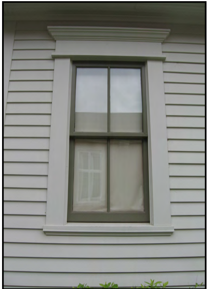
The two-over-two sash window at 619 Oak Street, NE, is an example of an appropriate modern wood sash window.
