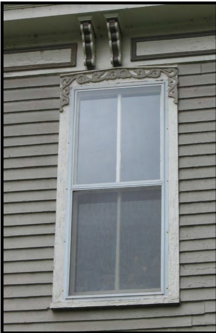
By the late nineteenth century, two-over-two wood sash windows were widely used in Decatur. Note: An appropriate storm window with a matching meeting rail has been added for energy conservation (618 Line Street, NE).
