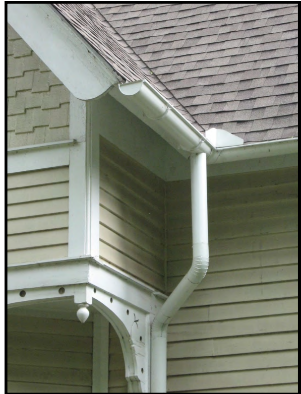
Gutters are recommended to be half-round design with round downspouts, (1006 Gordon Drive, SE, left and 305 Lafayette Street, NE, right).
