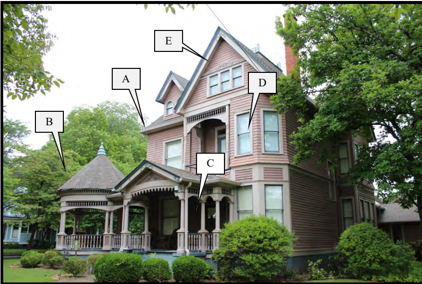
The Queen Anne style dwelling at 601 Ferry Street, NE, features an asymmetrical plan and wrap-around porch.
