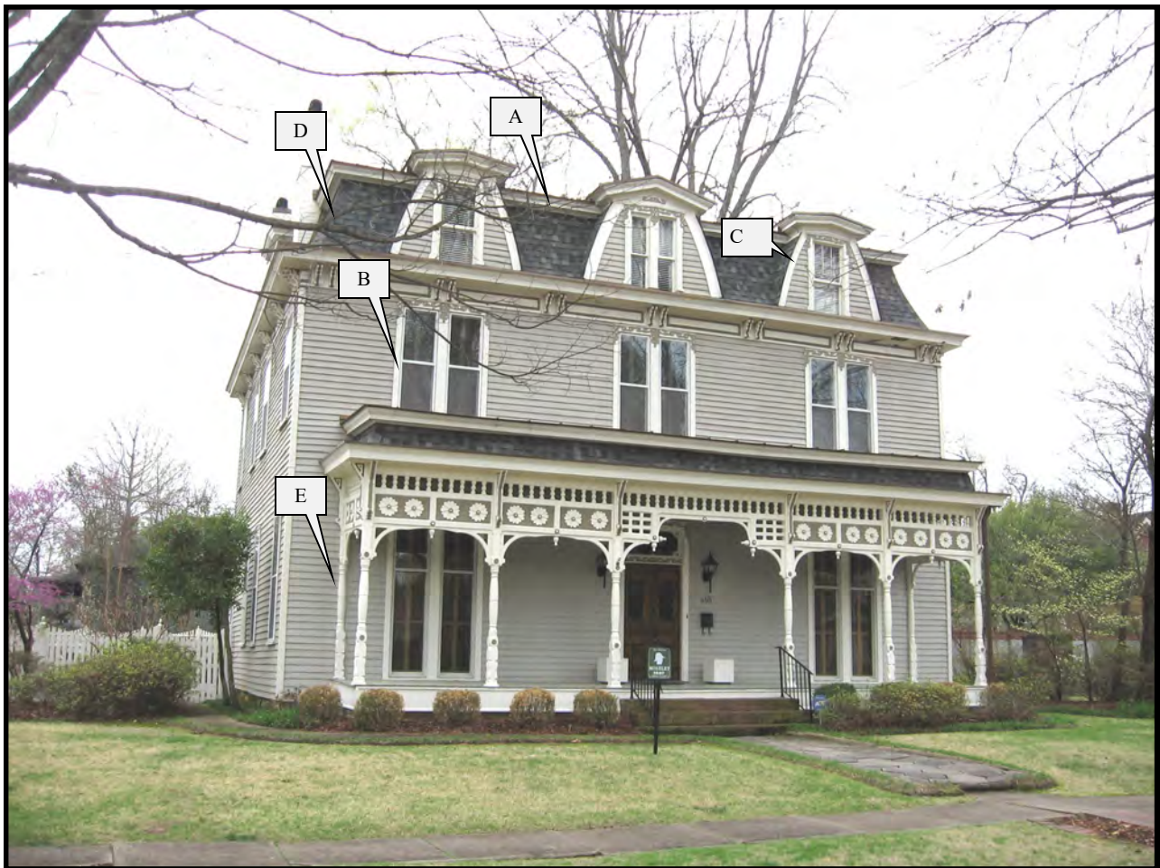
The Second Empire dwelling at 618 Line Street, NE, features the style's signature Mansard roof.
