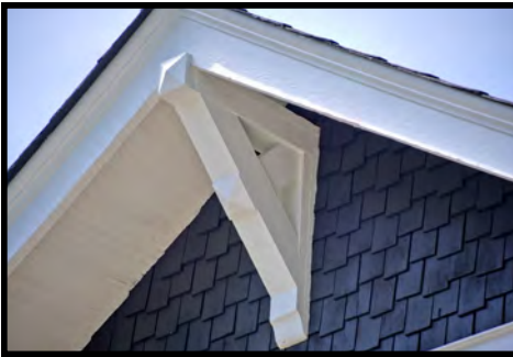
A common architectural detail on Craftsman dwellings are knee brace brackets at the eaves (804 Jackson Street, SE).
