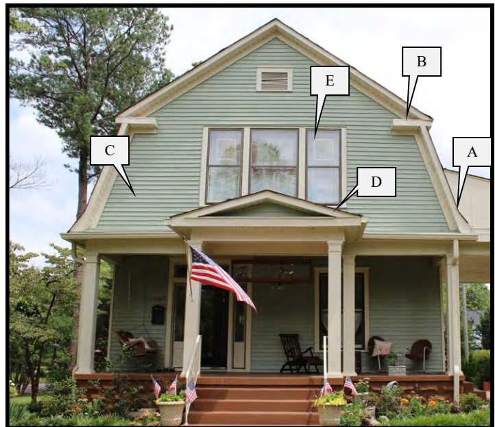
The dwelling at 1002 Sherman Street, SE, was designed with the gambrel roof facing the street and a full-width porch.
