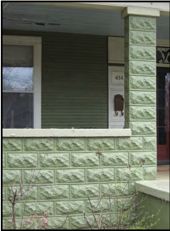
Rustic or rock-faced concrete block was used as an exterior wall material on dwellings built in the early 1900s (left, 414 Oak Street, NE; below, 503 Canal Street, NE).
