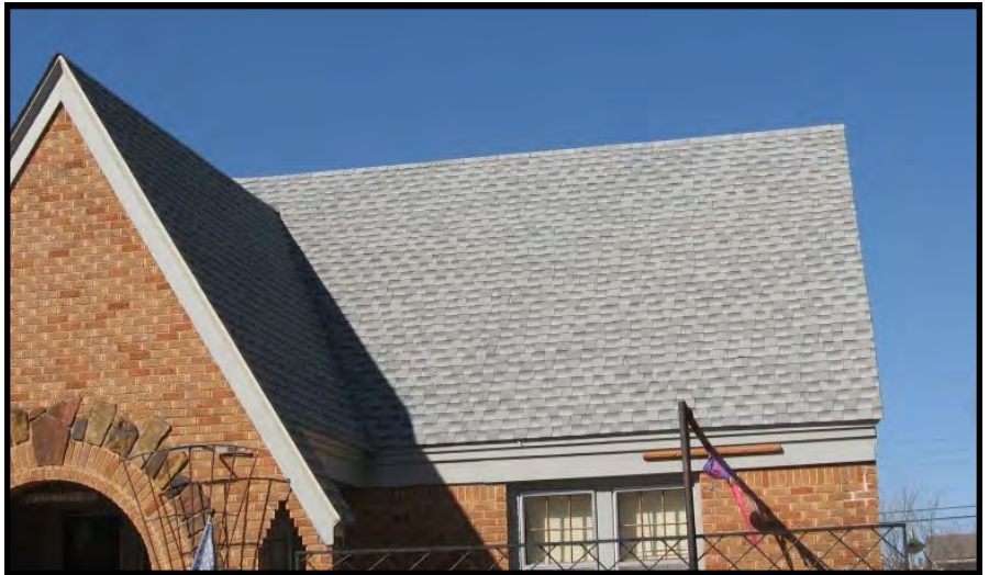
Reflective roof shingles may be appropriate for some dwellings. These assist in lowering cooling costs in warmer months.
