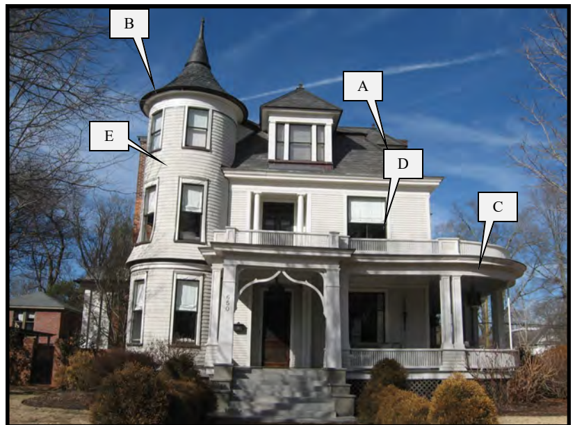
The dwelling at 650 Jackson Street, SE, displays a wraparound porch and a three-story corner tower.
