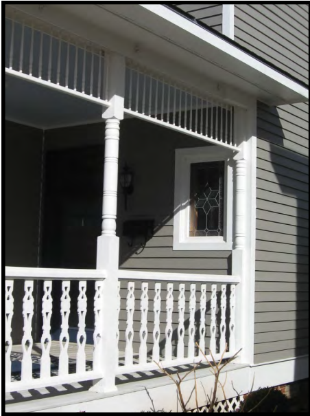
Victorian-era houses typically displayed milled porch columns with milled railings and frieze as at 408 4th Avenue, SE.
