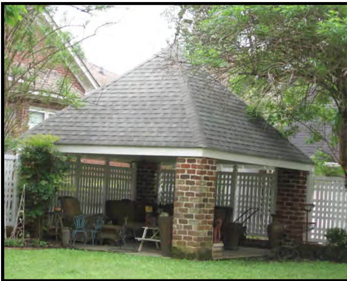
The gazebo at 622 Canal Street, NE, is appropriately sited in the rear yard.
