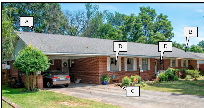
The Ranch style dwelling at 804 Johnston Street, SE, features a wide horizontal design, minimal decoration and attached carport.
