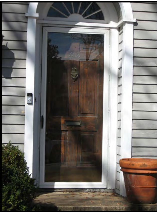
YES- Storm doors should be unobtrusive and blend with the historic door (403 Canal Street, NE).
