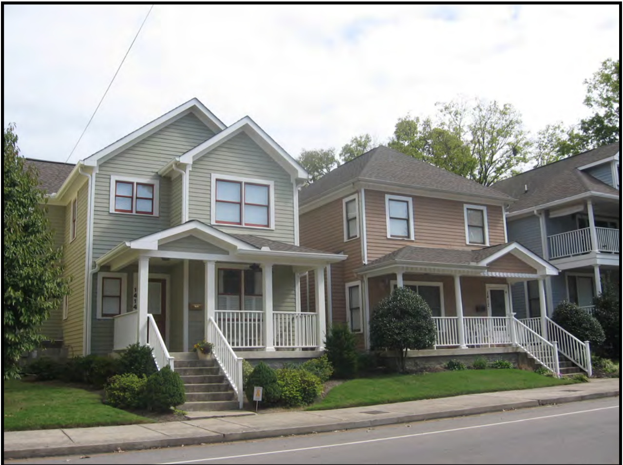
These new dwellings reflect traditional design elements common to the historic district. They have appropriate roof forms, porches on the main façade, consistent foundation heights and wood siding materials.
