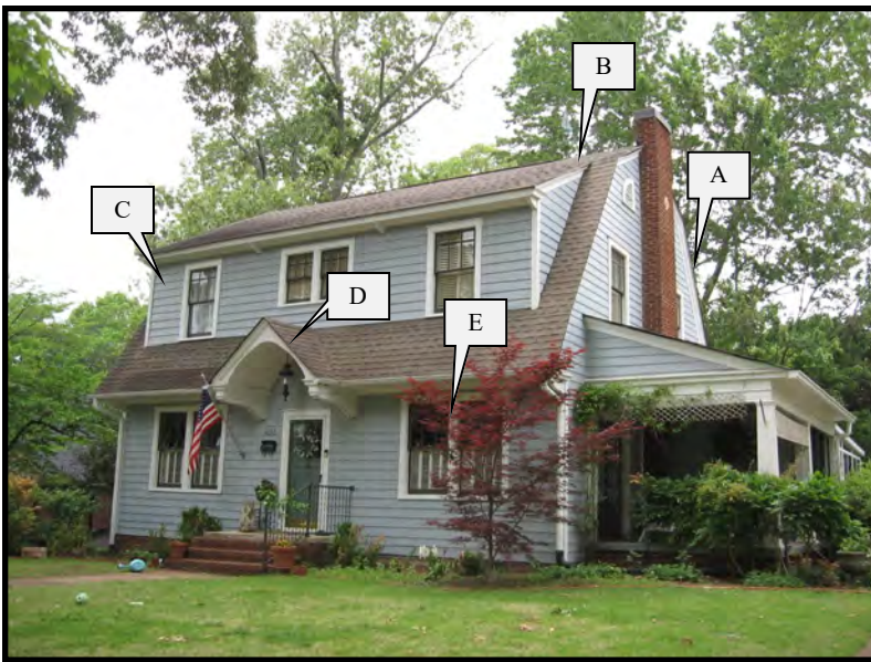
The Dutch Colonial style dwelling at 1036 Jackson Street, SE, has a gable roof stoop at the entrance and a side porch.
