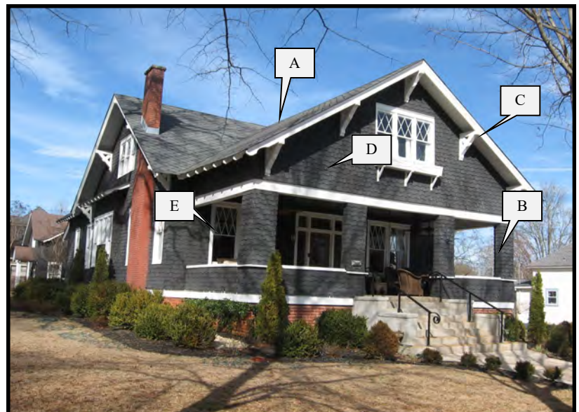
The Craftsman dwelling at 804 Jackson Street, SE, has a deep, full-width porch and knee brace brackets at the eaves.
