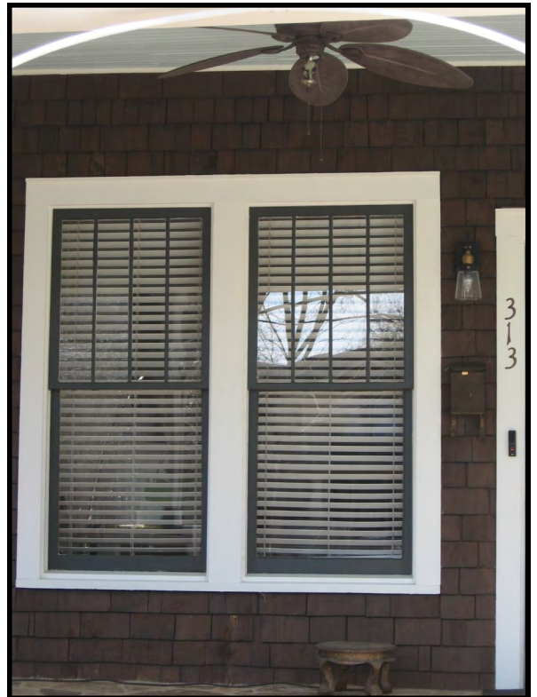
Many Craftsman-style dwellings were designed with vertical lights in the upper sash (313 Canal Street, NE).
