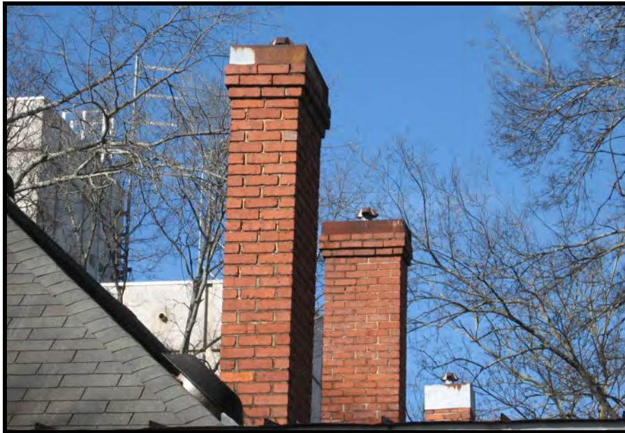
Corbelled brick is a common feature of chimneys on dwellings from the late nineteenth and early twentieth centuries (422 Jackson Street, SE).
