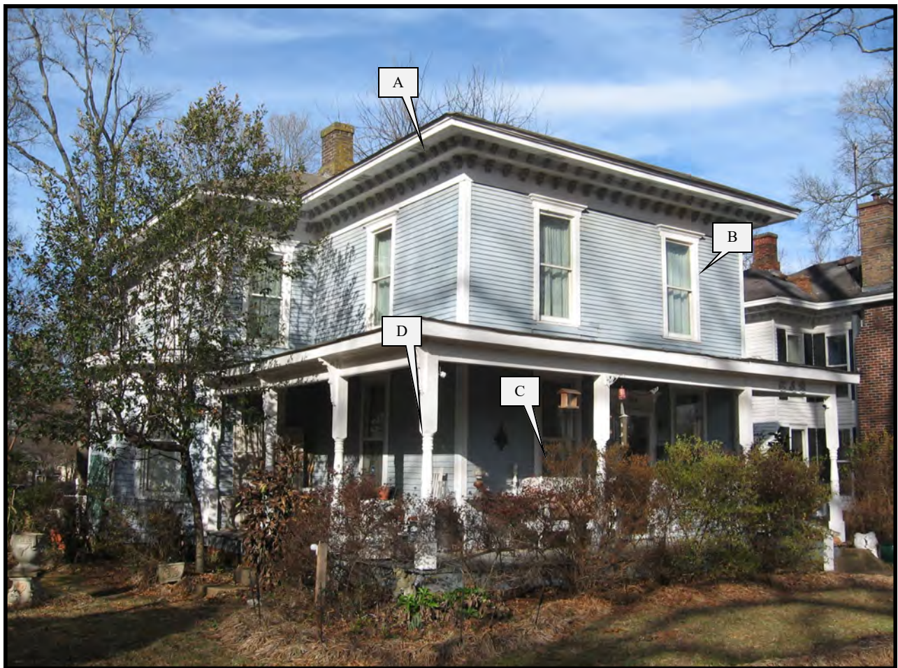
The Italianate style is represented in the dwelling at 648 Johnston Street, SE. Stylistic details include a cornice at the roofline, milled wood porch posts, an off-center entrance, window hoods, and eave brackets.
