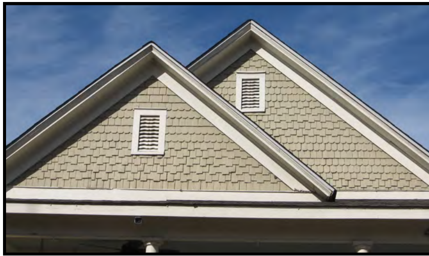
Wood shingles help date and define the architectural style of a dwelling (440 Sherman Street, SE).
