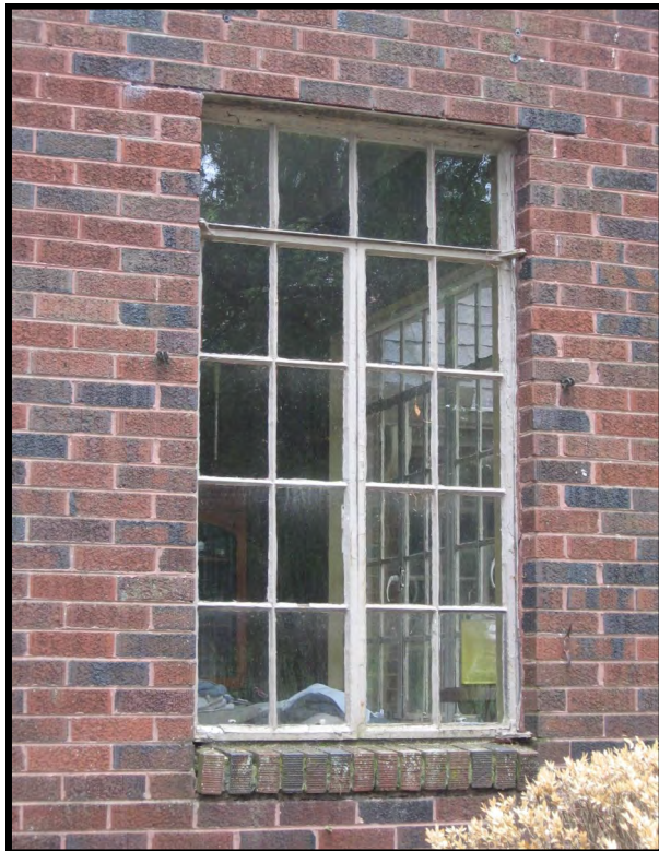
Steel casement windows were widely used for Tudor Revival-style dwellings in the early twentieth century (422 Oak Street, NE).
