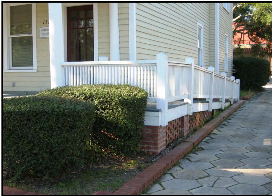
Examples of appropriately designed ADA ramps on the side (above) and front (below) of dwellings converted to commercial use. The railings reflect the original porch design and are screened by landscaping.
