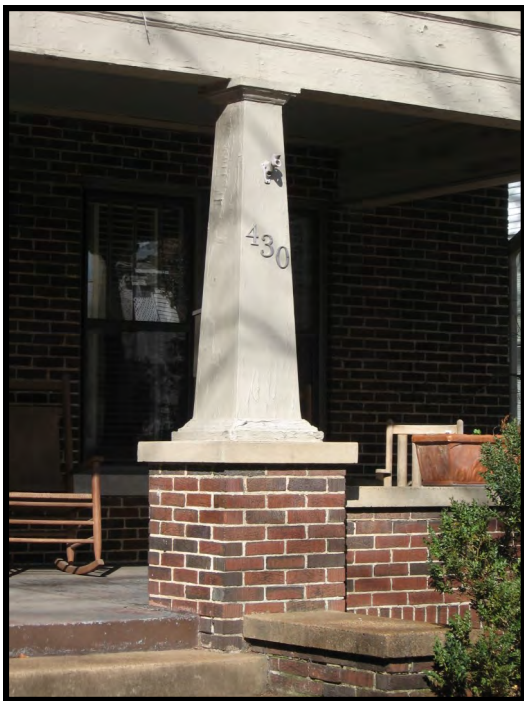
Tapered, wood posts on brick piers are common porch column designs on Craftsman dwellings as at 430 Jackson Street, SE.
