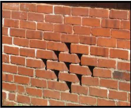
Brick foundation at 440 Sherman Street, SE.
