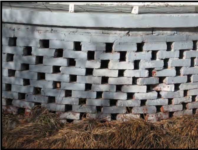
Piered brick foundation at 806 Grant Street, SE.
