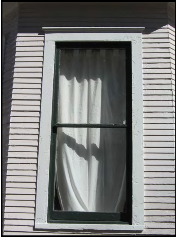
By the early twentieth century, one-over-one wood sash windows were the most common window designs in Decatur (701 Line Street, NE).
