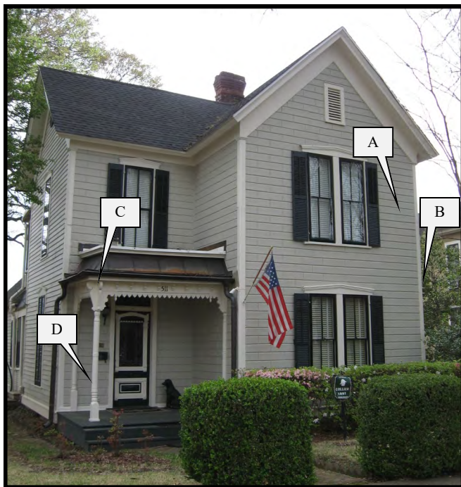
Two-story gabled ell plan dwelling at 513 Line Street, NE.
