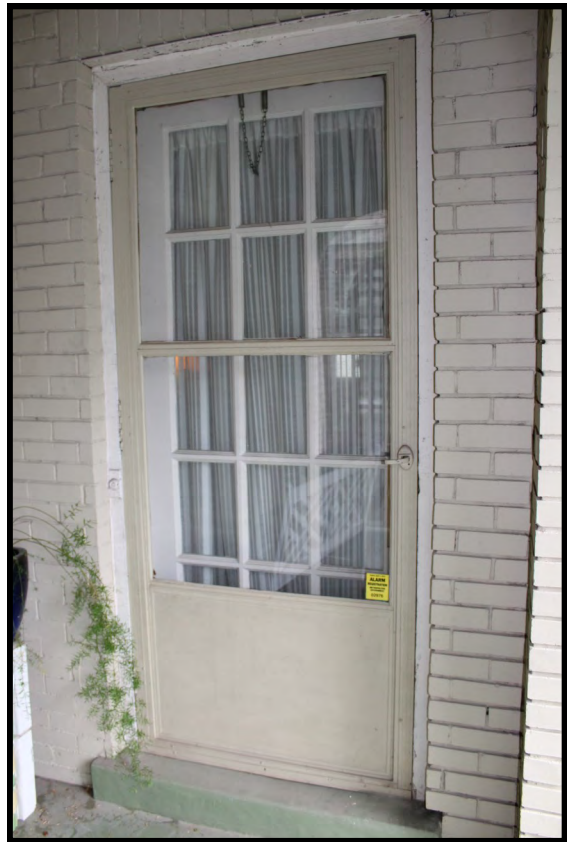
NO: Storm doors should be full-view to allow the historic door to be viewed behind it.
