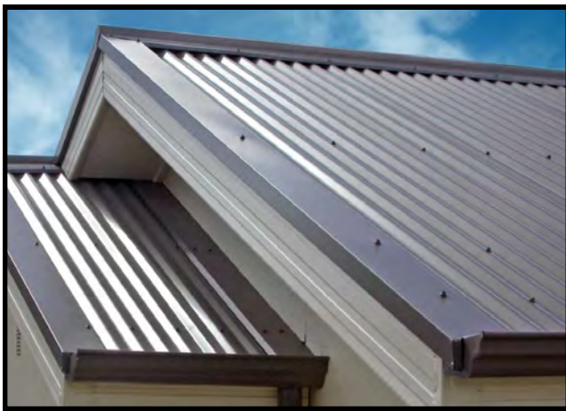
NO —Metal roofs which do not have traditional standing seam profiles and spacing are not appropriate.
