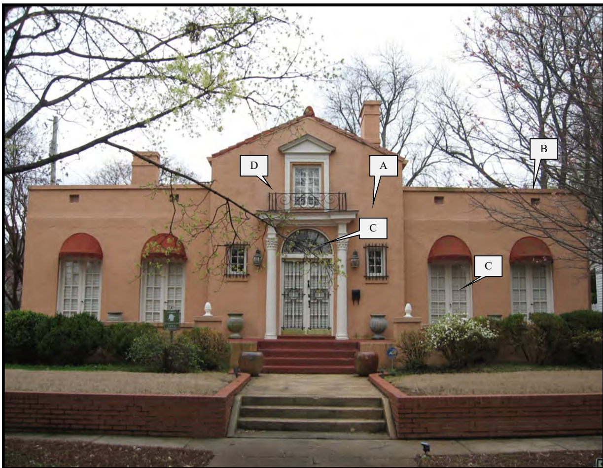
The Spanish Revival dwelling at 520 Line Street, NE, has a stucco exterior, clay tile roof, and rounded arched openings.
