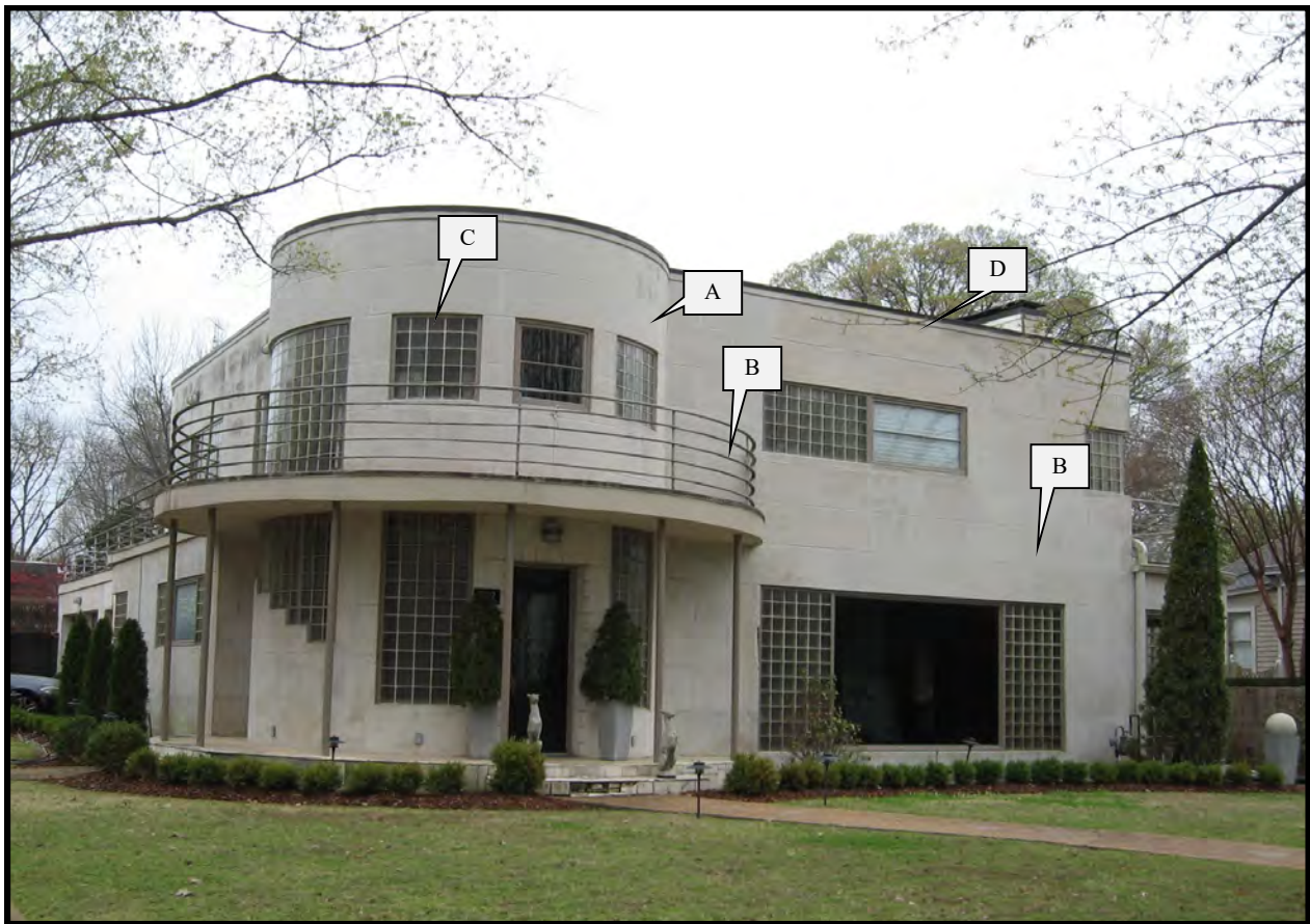
The Art Moderne style dwelling at 522 Oak Street, NE, is notable for its use of structural glass blocks, corner tower and stucco exterior.
