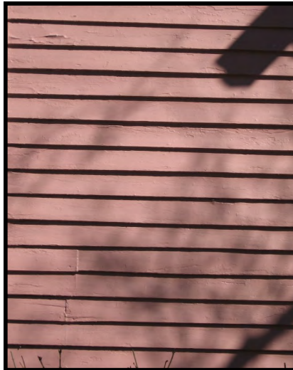
Preserve and maintain original wood siding materials. Clapboard siding is the most common wood siding material in the overlay district (left, 802 Gordon Drive, SE, and center, 503 Canal Street, NE). An unusual material is the rusticated wood siding designed to resemble stone blocks (right, 513 Line Street, NE).
