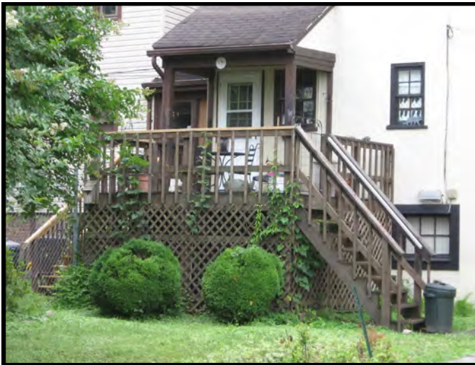
YES: Built at the rear of the dwelling, this deck is recessed from the side of the house and is appropriately scaled.
